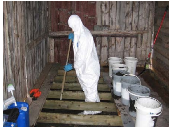
Excavation of mercury-contaminated soil at Kenai NWR
